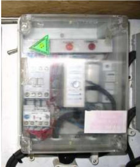
The water pump is in the generator shed. The green light will be on if the pump is bringing water up from the borehole. It takes about 20 minutes for the pump to fill the supply tank for the house.
