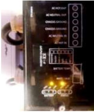
The solar power is controlled by the Inverter. Big black box on right. Both lights should be green when at optimal Left light shows the status of the stored power in the batteries: Full (green), OK (yellow), Low (red). If low run the generator.
